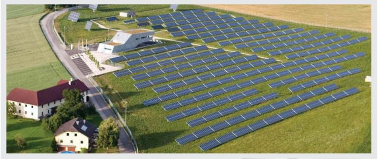
The 1MW PV system in Eberstalzell, Austria was built by energy supplier ENERGIE AG not just as a power plant, but also as a research station with the purpose of measuring the yield, service life and degradation of a range of different PV modules.
